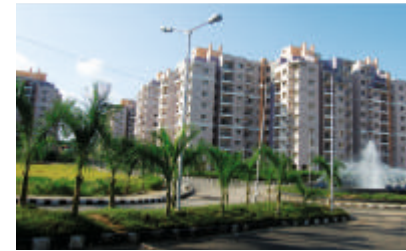
NCC Khelgaon, Hotwar
